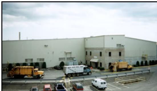
The Facility had three (3) modular mass-burn refractory lined combustors, each rated at 136 tons per day of MSW. Each combustor had an associated waste heat boiler, rated at 31,528 pound per hour of steam, and a state-of-the-art air quality control system (AQCS). The Facility also had a 9.46 mw condensing turbine generator.
