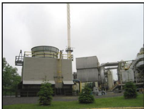
In each municipal waste combustor 'train,' flue gas flowed from a primary chamber into a secondary chamber, where sufficient time and temperature were provided to assure complete combustion. From the secondary chamber, flue gas flowed into a tertiary chamber, then into the heat recovery and air quality control systems.
